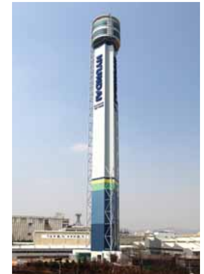
The tallest elevator test tower(Hyundai Asan Tower) stands in Icheon, Korea.
